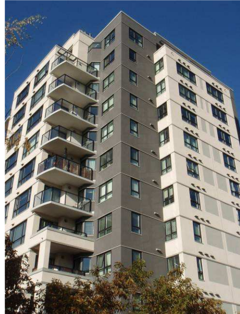
Admiral Point, Vancouver, BC – After rehabilitation
