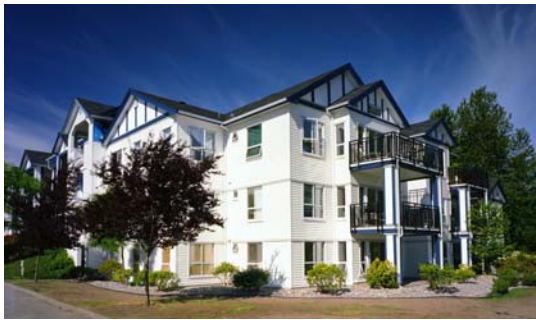
The Shorewalk, Ladner, BC - full building enclosure rehabilitation
