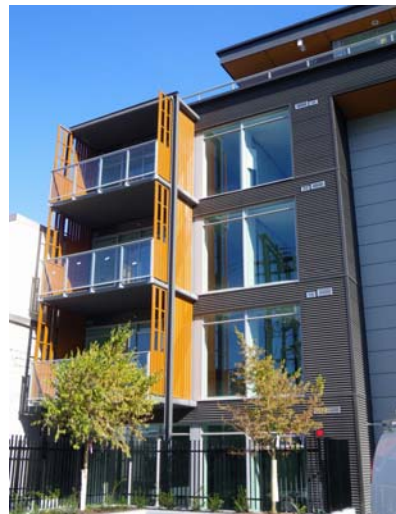
Jacobsen, Vancouver, BC - steel frame construction
