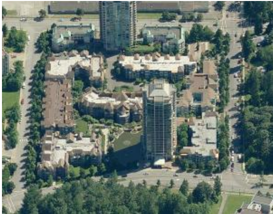
Lakeside Terrace, Coquitlam, BC
