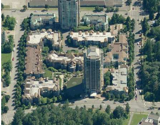
Lakeside Terrace, Coquitlam, BC
