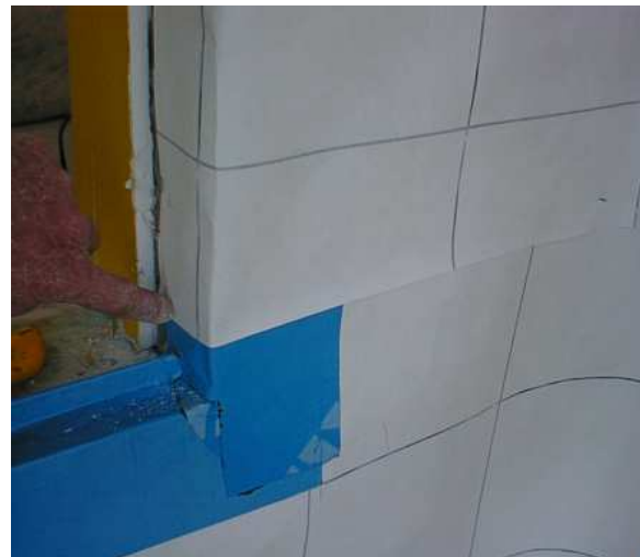
Appropriate use of membrane at window sill and jamb
