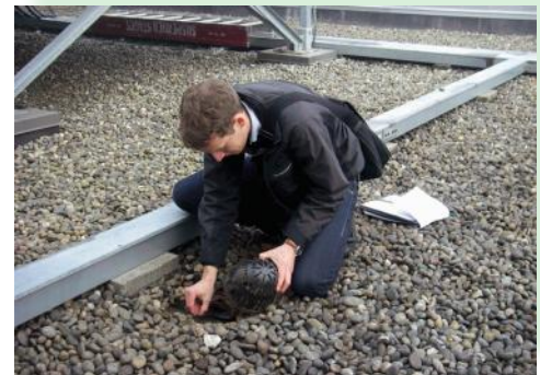
Roof drain cleaning
