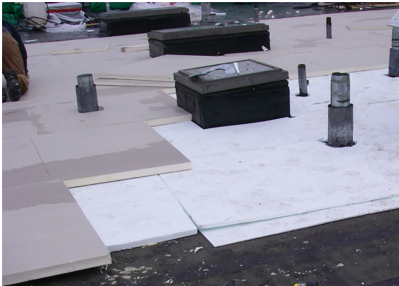
Figure 1: Tapered EPS insulation below polyisocyanurate insulation in a low slope roof application.
